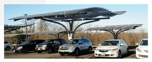
Sigma had performed a simulated hurricane wind analysis to better determine wind-induced loads. The firm studied and used this data to update various structural components, which improved the arbor's ability to withstand 120 mph hurricane winds.
